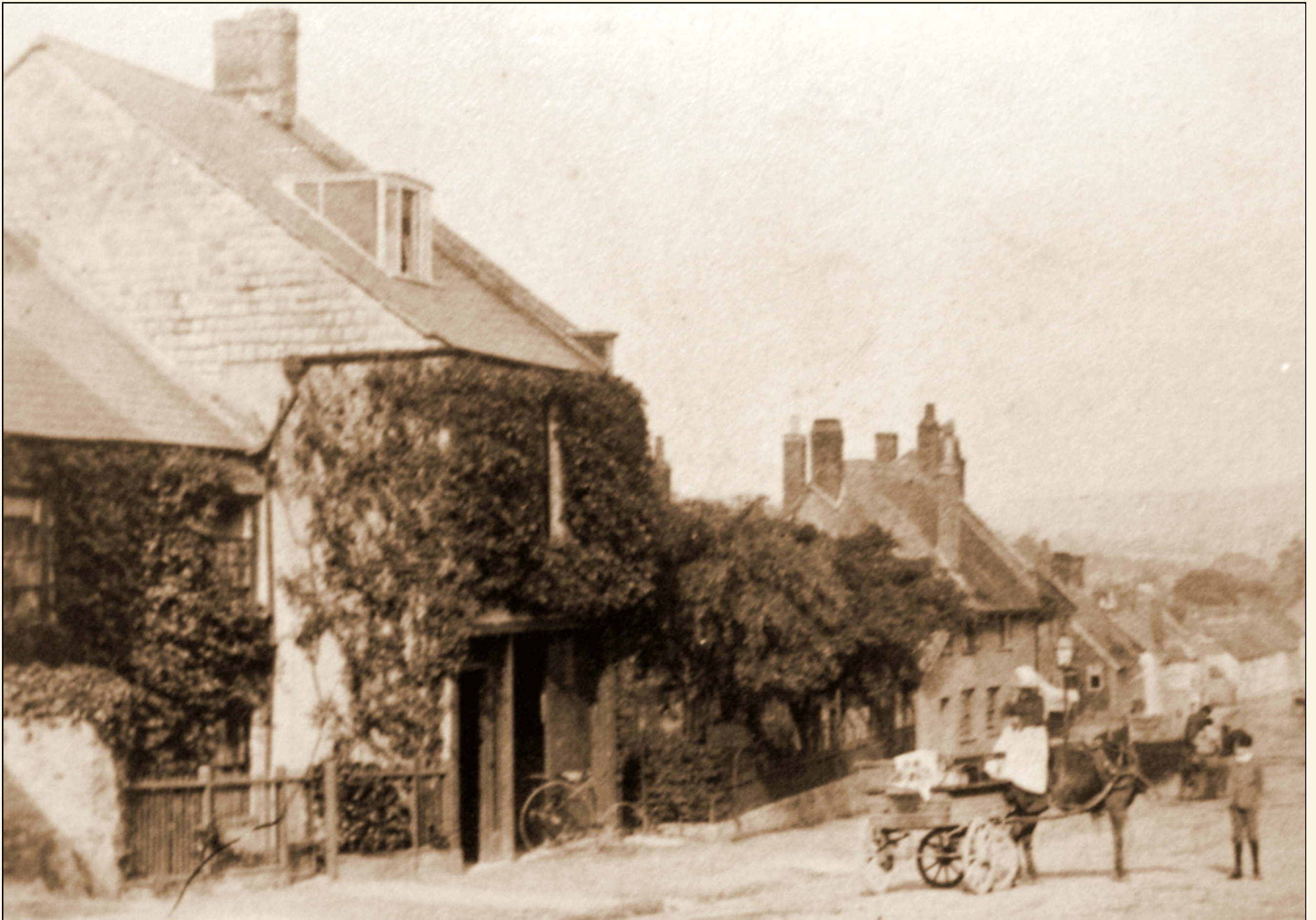
Pre 1894 View looking down the Street with Little Lodge on the left
